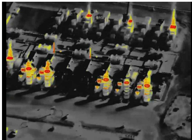
Figure 2. Thermal camera image of xAI's Stanton Road S. facility (Oct. 31, 2025; Steve Jones/SouthWings).
