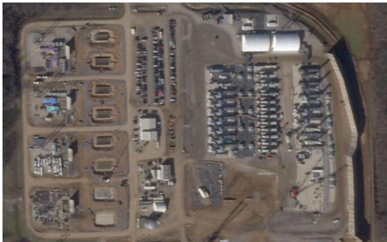
Figure 3. Close-up aerial image of xAI’s Stanton Road S. facility showing 27 turbines (Feb. 9, 2026).
